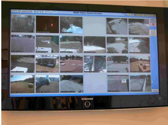
Figure 2: This screen shows up to 24 still images from remote sites at one time. Each image is updated every 20 minutes. If an alarm occurs, the operator receives a 15-second video clip of the incident and can switch to live video at any time.
