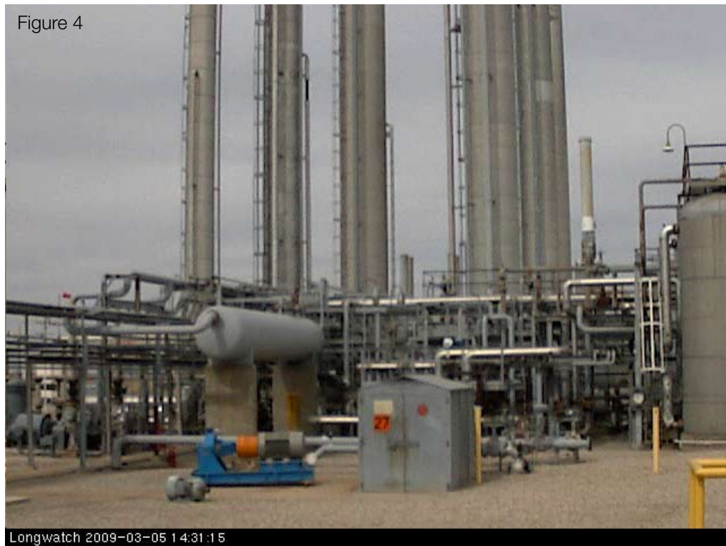
Figure 4: The operator can request that archived DVR data be transmitted to the control room at any time, or it can be downloaded to a thumbdrive or portable hard drive and brought to the control room.
