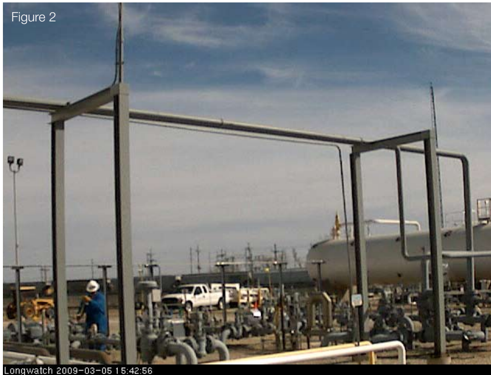
Figure 2: Live video is sent to the control room via the 42KB/sec wireless link. With Longwatch, the wireless system supports three cameras. Each camera requires 13KB/sec, so the network supports three live cameras while it archives video from all four cameras.
